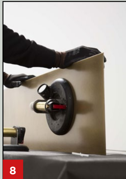
Use one/two suction cups to lift the slab and apply it on the substrate.
