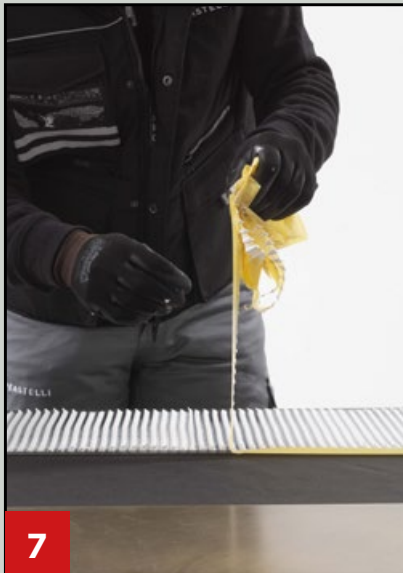
Remove the adhesive tape for wall application.
